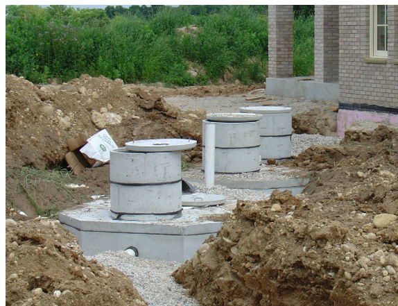
Washington County regulates POWTS for any development in the County that is not served by a public sanitary sewer system.
