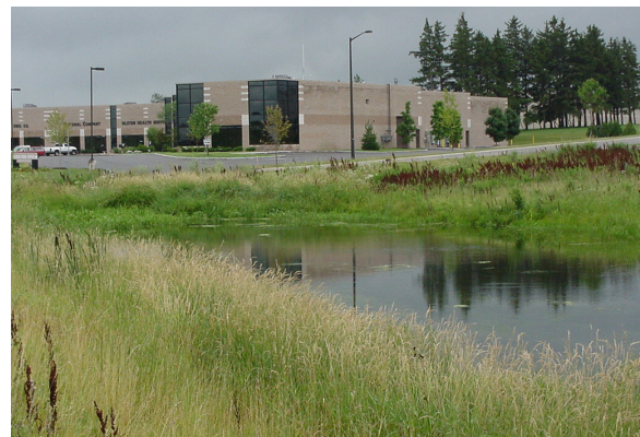
Detention basins are designed to accommodate stormwater runoff.
