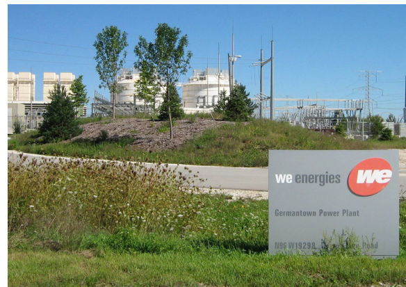
Most of Washington County is provided with electric power service by We Energies.
